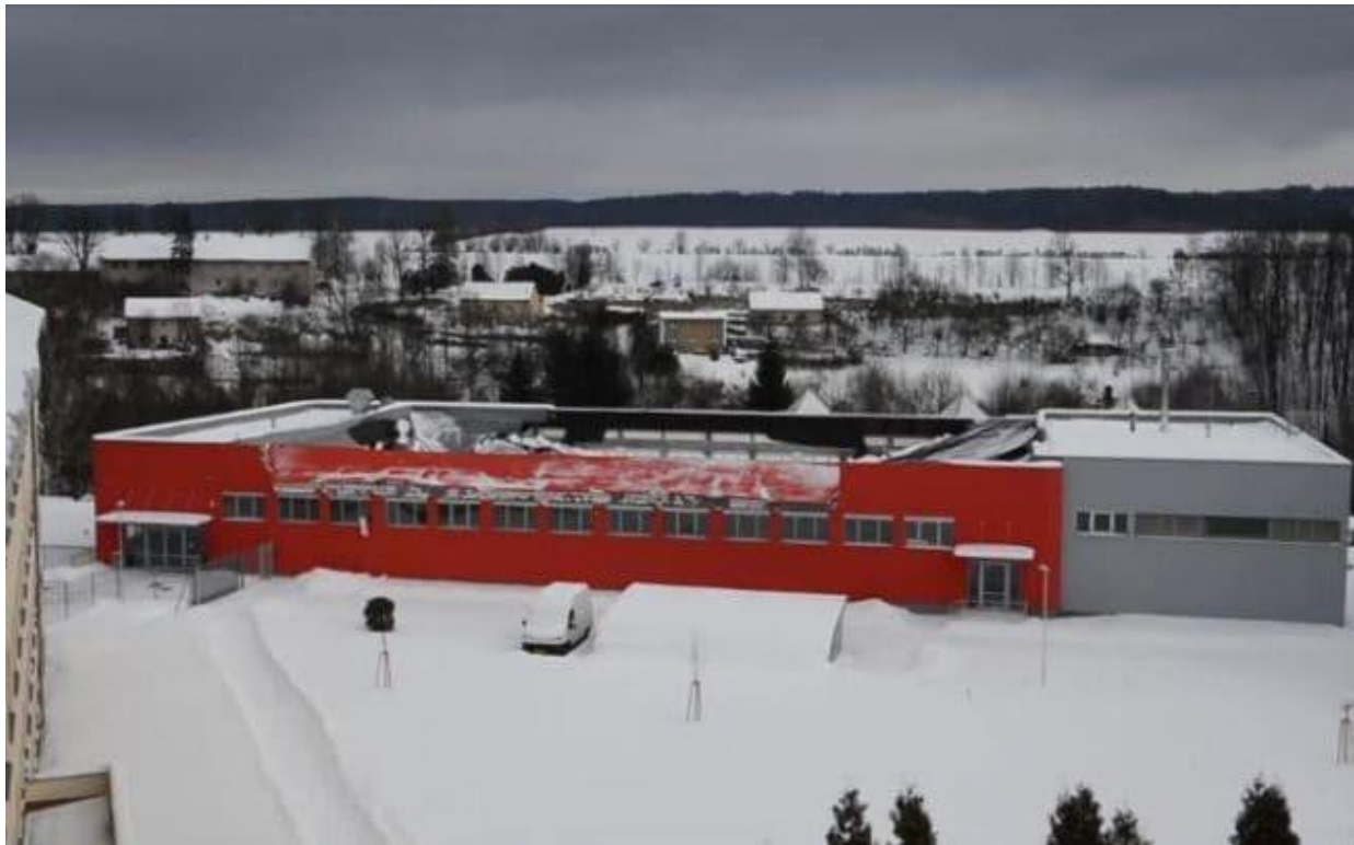
Figure 3: Česká Třebová Sports Hall After the Collapse of the Roof 19
